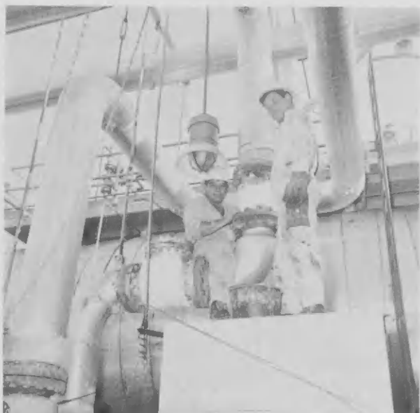
While Pipestill No. 5 is down for turnaround, Lindoro Hernandez and Jacobo Ridderstaat apply blanket-type insulation on bare fittings.
